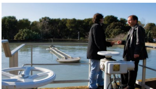
Water and Wastewater Treatment
